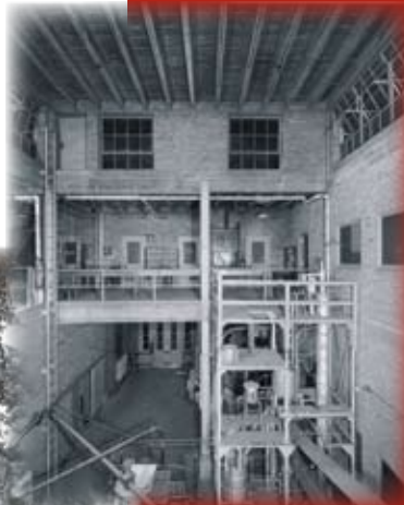
A packed column inside original Sweeney Hall
